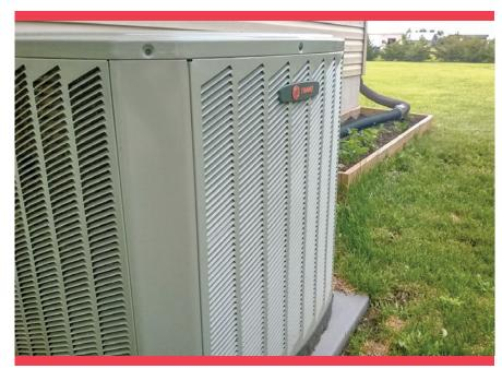
Heat pump systems located outside a home should be cleaned twice a year – in the spring and fall. In addition, be certain to check electrical connections annually and replace or righted as needed.
