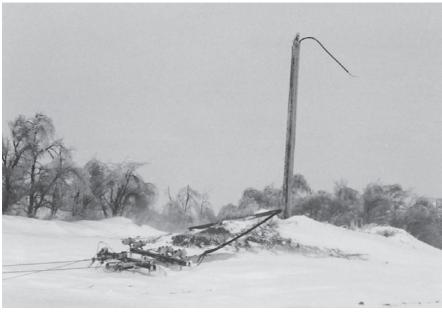
The weight of ice on power lines and poles can cause them to snap. Electric cooperatives try to be prepared for weather events that could cause damage. While costly, long-term weather extremes can enter into electric rates even more so than short-term weather extremes.
