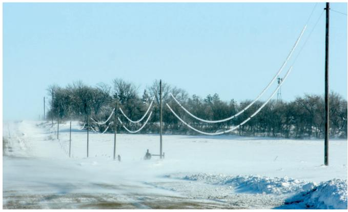
The sagging electric wires could bring power outages if wind starts the line to gallop and bounce so wires touch.
