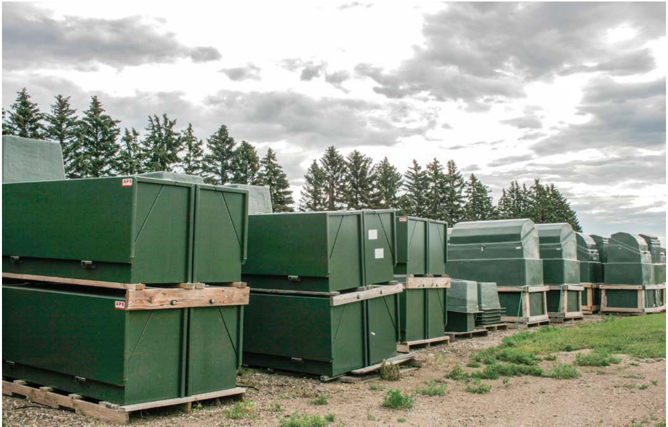
Several underground cabinets and enclosures in McLean Electric Cooperative's materials yard in preparation for 2022 construction.
